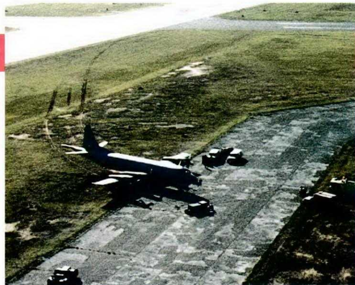
"Overview of the occurrence site looking west toward the threshold of Runway 11."
